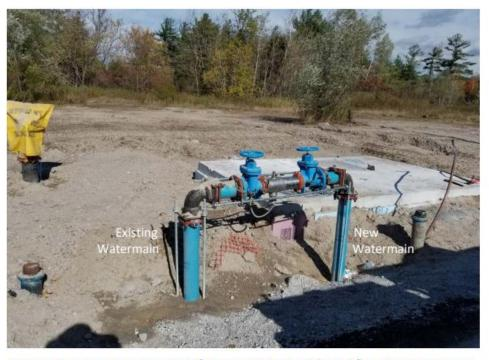
Figure A-2: Temporary connection from a watermain with *Backflow Prevention* using a CSA-certified reduced pressure principle backflow preventer.
