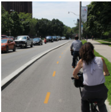
Two-Way Bicycle Lane Separated by Cast-in-place Concrete Curb, Toronto
