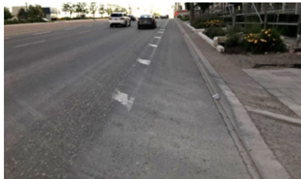
Figure 10.14 – Worn Bicycle Pavement Markings
