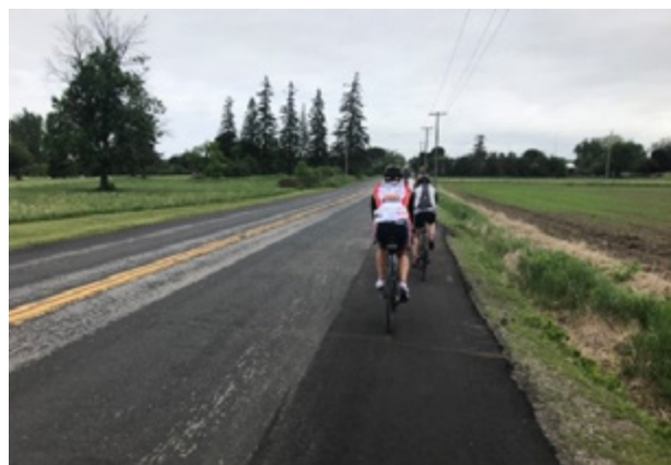
Figure 8.14 – Newly Resurfaced Paved Shoulders, York Region
