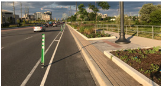
Figure 4.23 – Flex Bollard Separation, Markham
