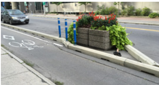
Figure 4.25 – Pre-cast Concrete Curb Separating a One-way Separated Bicycle Lane, Ottawa
