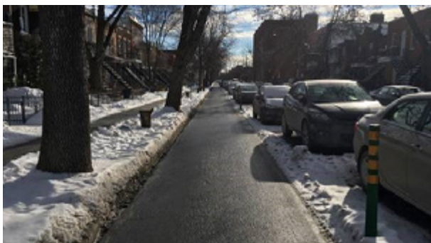
Figure 10.21 – Cycle Track Cleared by Sweeper with Brine Applied to Surface, Montreal
