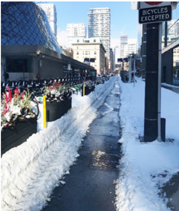
Figure 10.25 – Protected Bike Lane Cleared of Snow, Toronto
