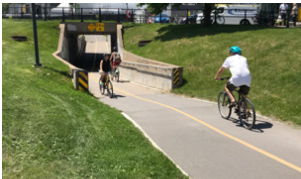
Figure 6.92 – Grade Separated Crossing, Montréal
