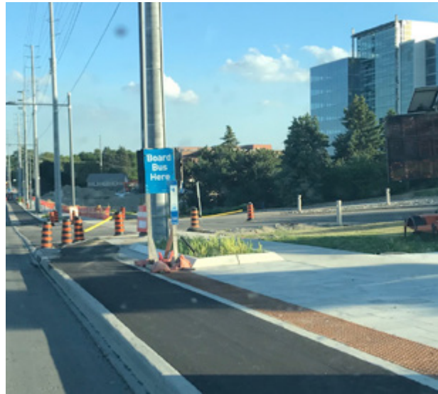
Figure 10.11 – Cycle Track Constructed with Concrete Base and Asphalt Surface, Newmarket
