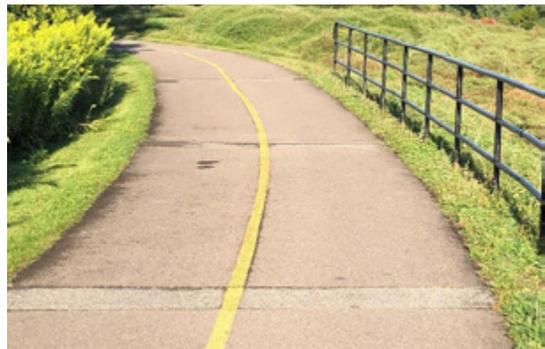
Figure 10.8 – Transverse Cracking
