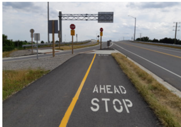
Figure 6.87 – Ramp Crossing, Cambridge
