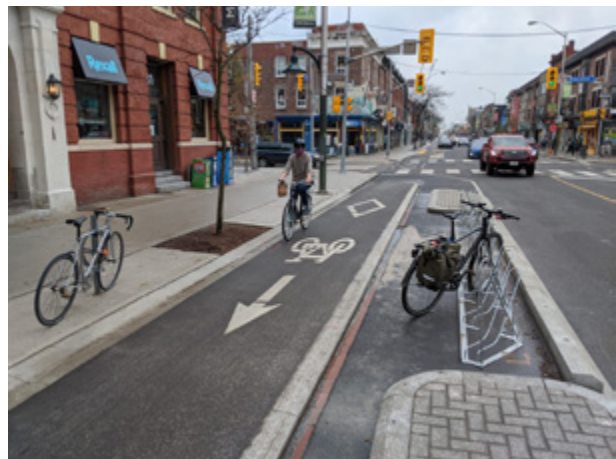
Figure 9.2 – On-Street Parking Corral, Toronto
