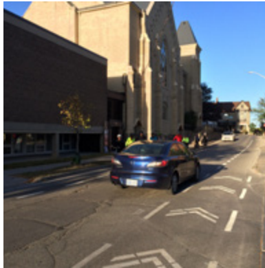
Advisory Bicycle Lane on Urban Street with No On-Street Parking, Newmarket
