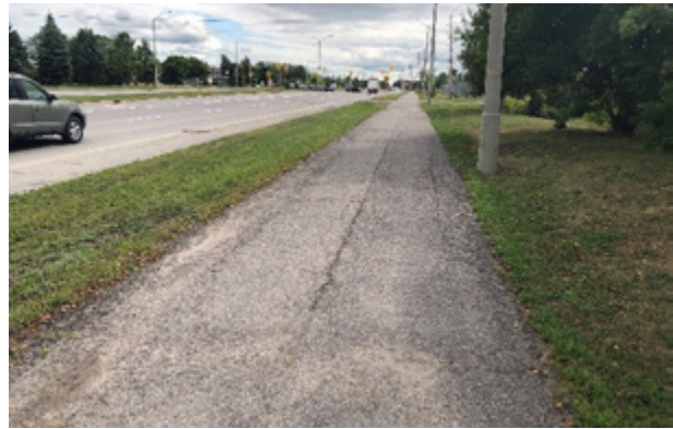
Figure 10.7 – Longitudinal Cracking
