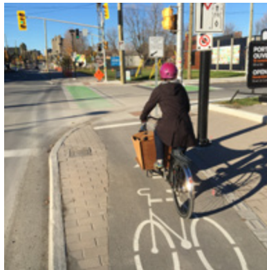
Cycle Track Separated by Barrier Curb, Ottawa
