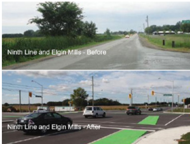
Figure 8.6 – Pre- and Post-construction Comparison
