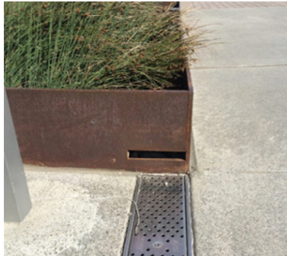
Figure 7.16 – Trench Drain at a Flush Surface
