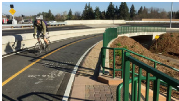
Figure 6.86 – Grade-separated Multi-use Path Through an Interchange, Sacramento, California
