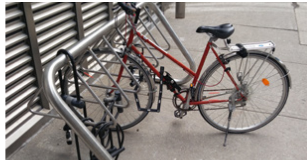
Figure 9.12 – Coat-hanger Rack (Not Preferred for Most Situations)
