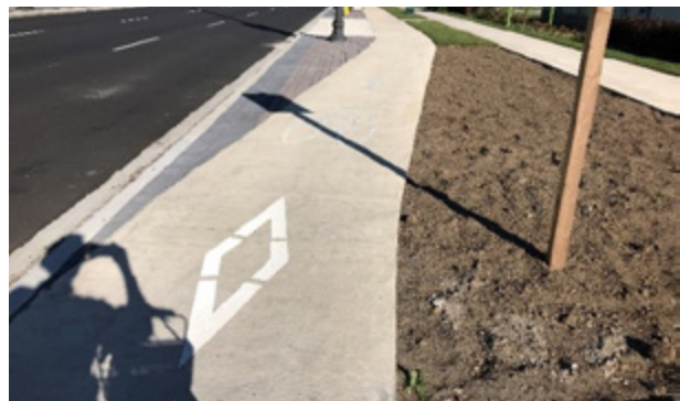
Figure 10.15 – Example of Markings on Concrete (Bicycle Symbol Not Visible)
