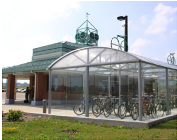
Figure 3.5 – Bike Parking at Commuter Rail Station, Markham
