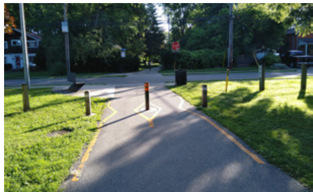
Figure 7.14 – Example of Bollards with Reflectors and Directional Edge Lines, Burlington
