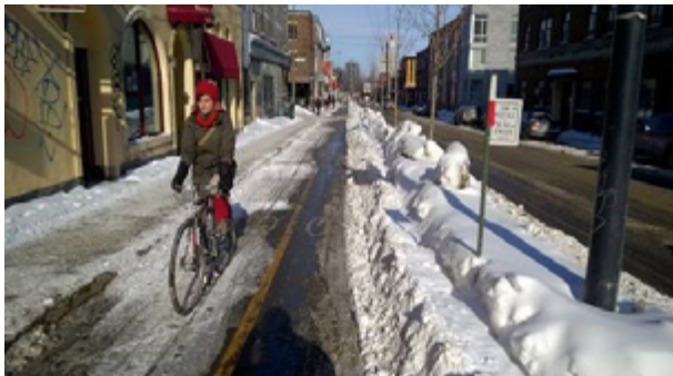
Figure 10.20 – Cycle Track Plowed with Salt Applied to Surface, Montreal
