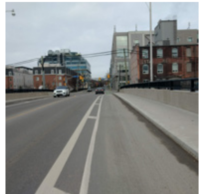
Buffered Bicycle Lane, Toronto
