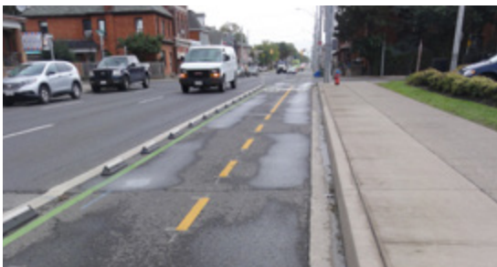
Figure 4.27 – Rubber Curb Separating a Two-way Separated Bicycle Lane, Hamilton
