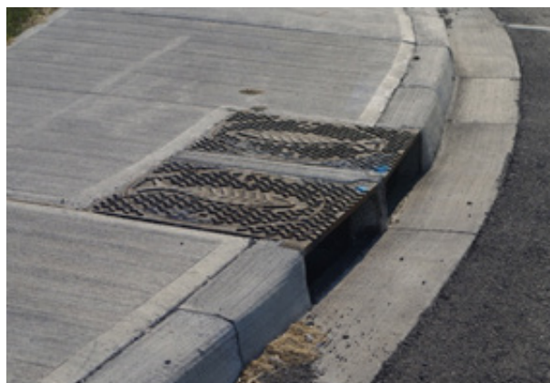
Figure 7.15 – Side-Inlet Catch Basin
