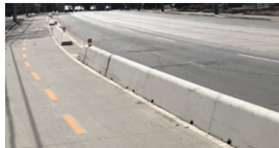
Figure 4.28 – Low Wall Concrete Barriers Separating a Two-way Separated Bicycle Lane, Toronto
