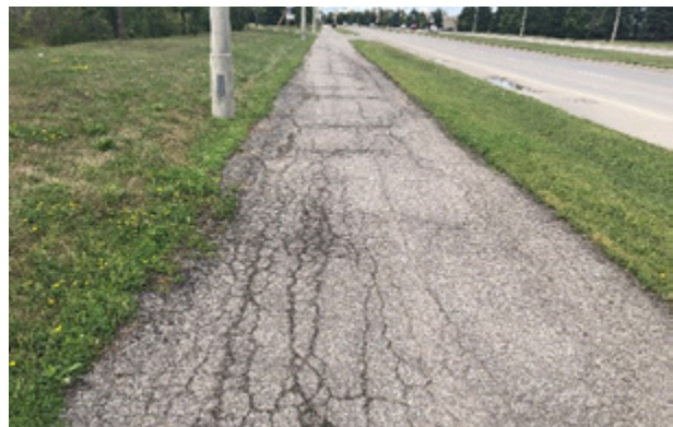
Figure 10.9 – Alligator Cracking
