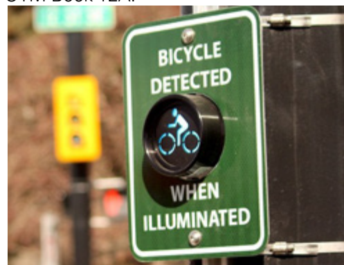
Figure 6.61 – Bicycle Detection Indicator, Calgary
