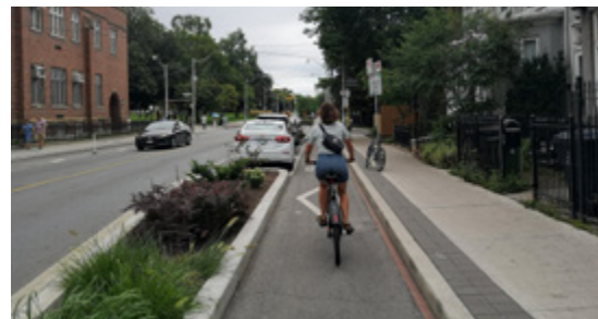
Figure 4.26 – Cast-in-place Concrete Curb Separating a One-way Separated Bicycle Lane, Toronto
