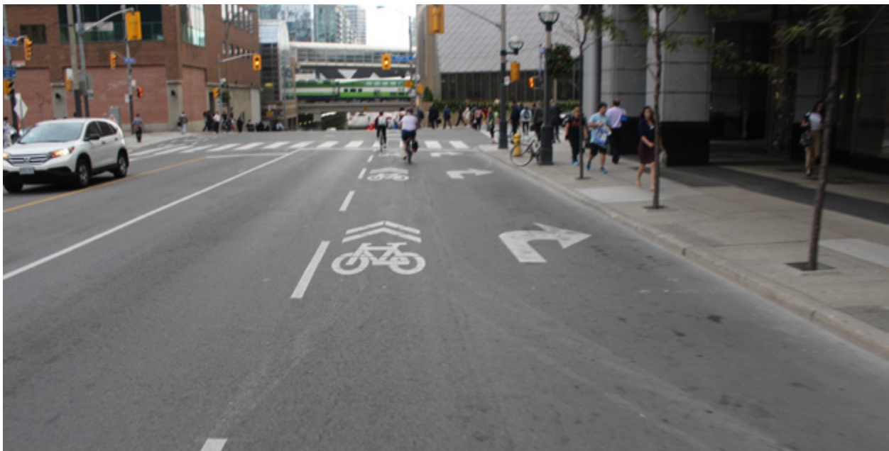
Figure 6.45 – Example of Mixing Zone, Toronto
