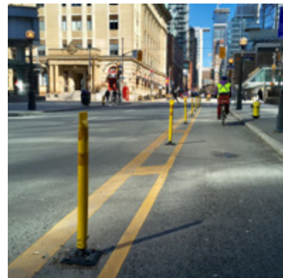
Contraflow Bicycle Lane Separated by Bollards, Toronto
