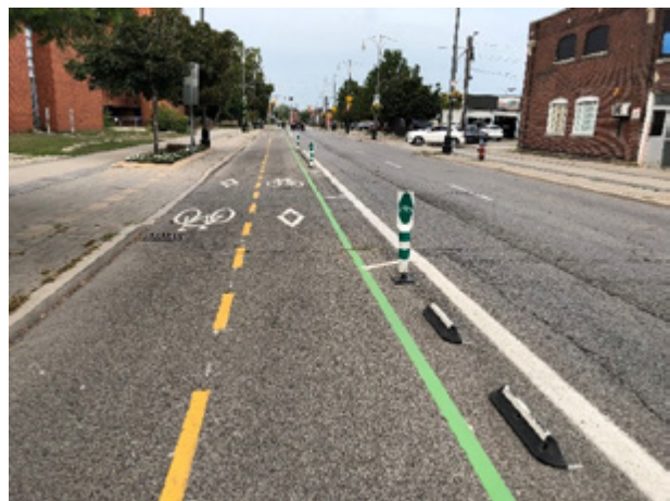
Figure 10.6 – Well-Maintained Cycling Facility, Hamilton
