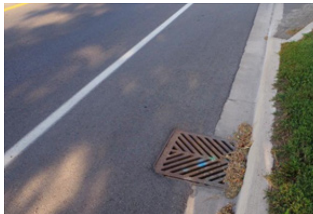
Figure 7.17 – Drainage Grate with Herringbone Openings
