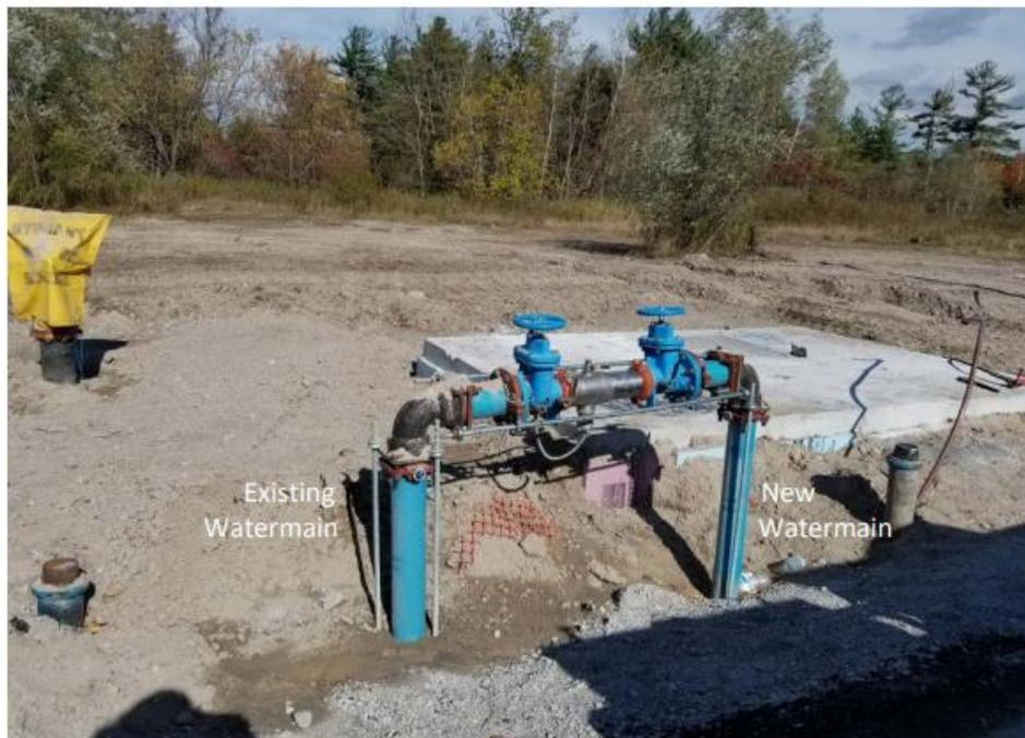
Figure A-2: Temporary connection from a watermain with *Backflow Prevention* using a CSA-certified reduced pressure principle backflow preventer.
