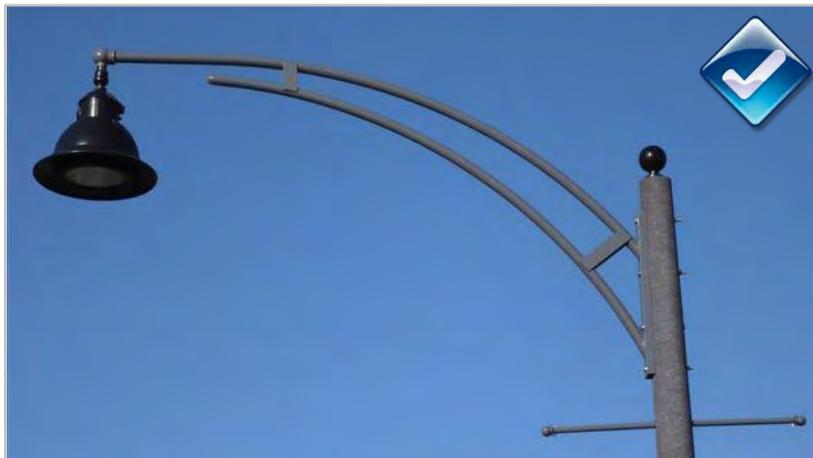
Figure 5: Full Cut-off Light Standard
