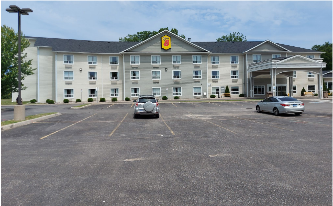
Figure 3 – Subject Site (Primary West Elevation) – Photo Taken by GWD Sunday July 2, 2023
