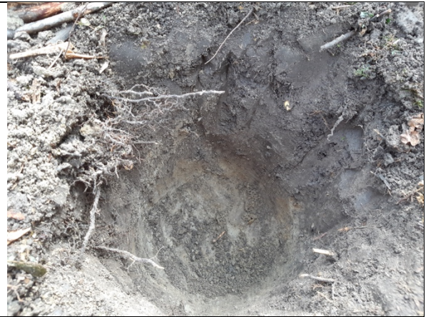
IMAGE 8 UNDISTURBED TEST PIT IN PROGRESS
