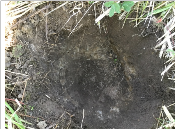
IMAGE 7 DISTURBED TEST PIT IN PROGRESS
