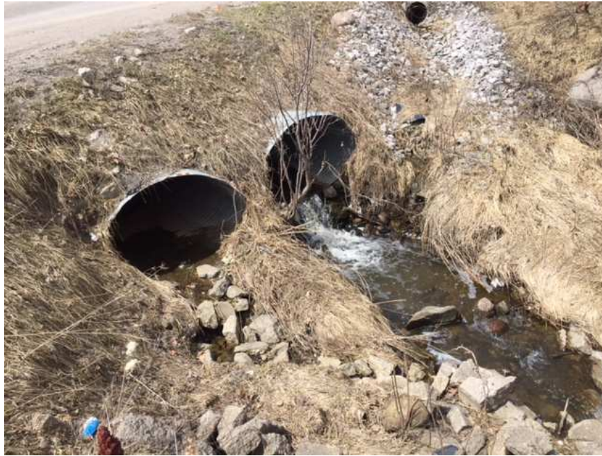
Photo 11. View of double culverts at outlet east of William St (April 27, 2018)
