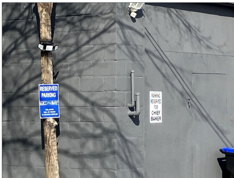
Photograph 14 – Observed fill/vent pipes at property located northeast of the Site (253 King Street).
