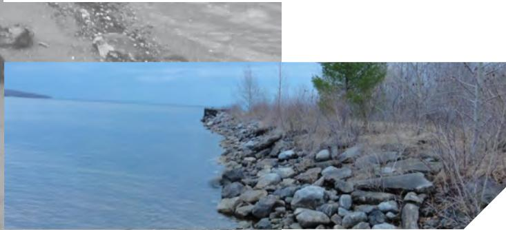
Ad hoc shore protection consisting of dumped concrete rubble, stone and asphalt. This shoreline could be developed as a series of headland/beaches.
