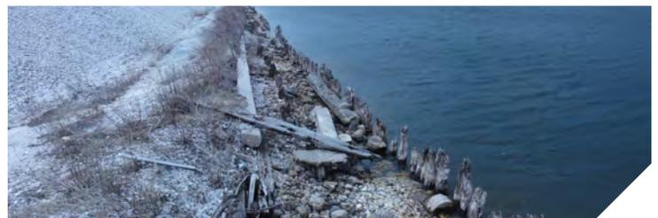
Failed timber wall at toe of steep bluff. A revetment or seawall would be suitable protection for this shoreline.
