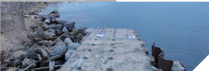
The SSP wall shown above has failed. A headland beach could be developed in this area. It should be noted that there is severe undermining under some of these slabs and that all of the stone material has been removed. The slabs are resting only on timber piles, which appear to be rotting. These piles will rot out and the slab will collapse.
