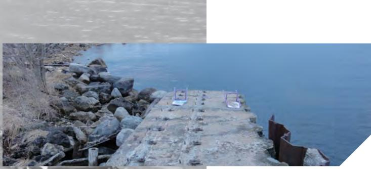
The SSP wall shown above has failed. A headland beach could be developed in this area. It should be noted that there is severe undermining under some of these slabs and that all of the stone material has been removed. The slabs are resting only on timber piles, which appear to be rotting. These piles will rot out and the slab will collapse.
