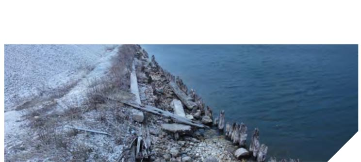
Failed timber wall at toe of steep bluff. A revetment or seawall would be suitable protection for this shoreline.
