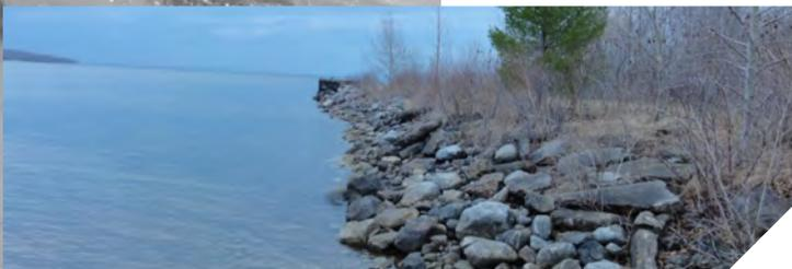
Ad hoc shore protection consisting of dumped concrete rubble, stone and asphalt. This shoreline could be developed as a series of headland/beaches.
