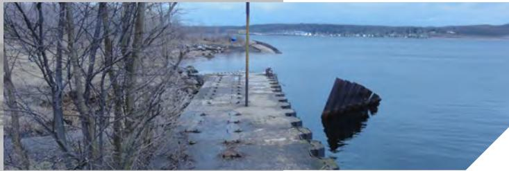
The SSP wall starts to fail a couple hundred meters along the wall. There are signs of undermining and the concrete has detached from the SSP. Some of the slabs have started to shift.
