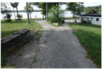
Figure 20: Asphalt roadway needing repair work
