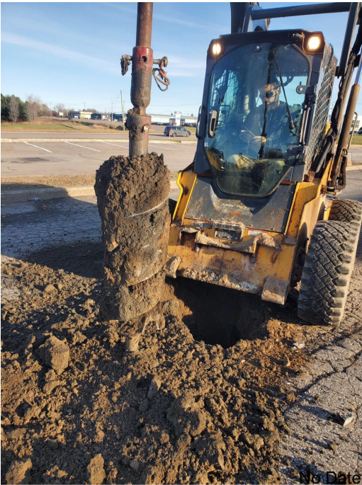
Augured drill holes.
